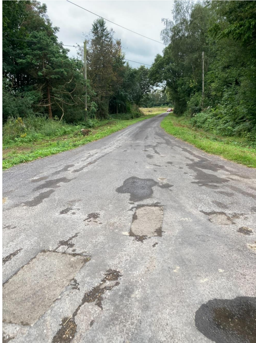
Figure 3 - looking westwards along Knoll Farm Road towards the application site
